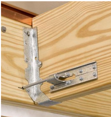
Deck Tension Ties
